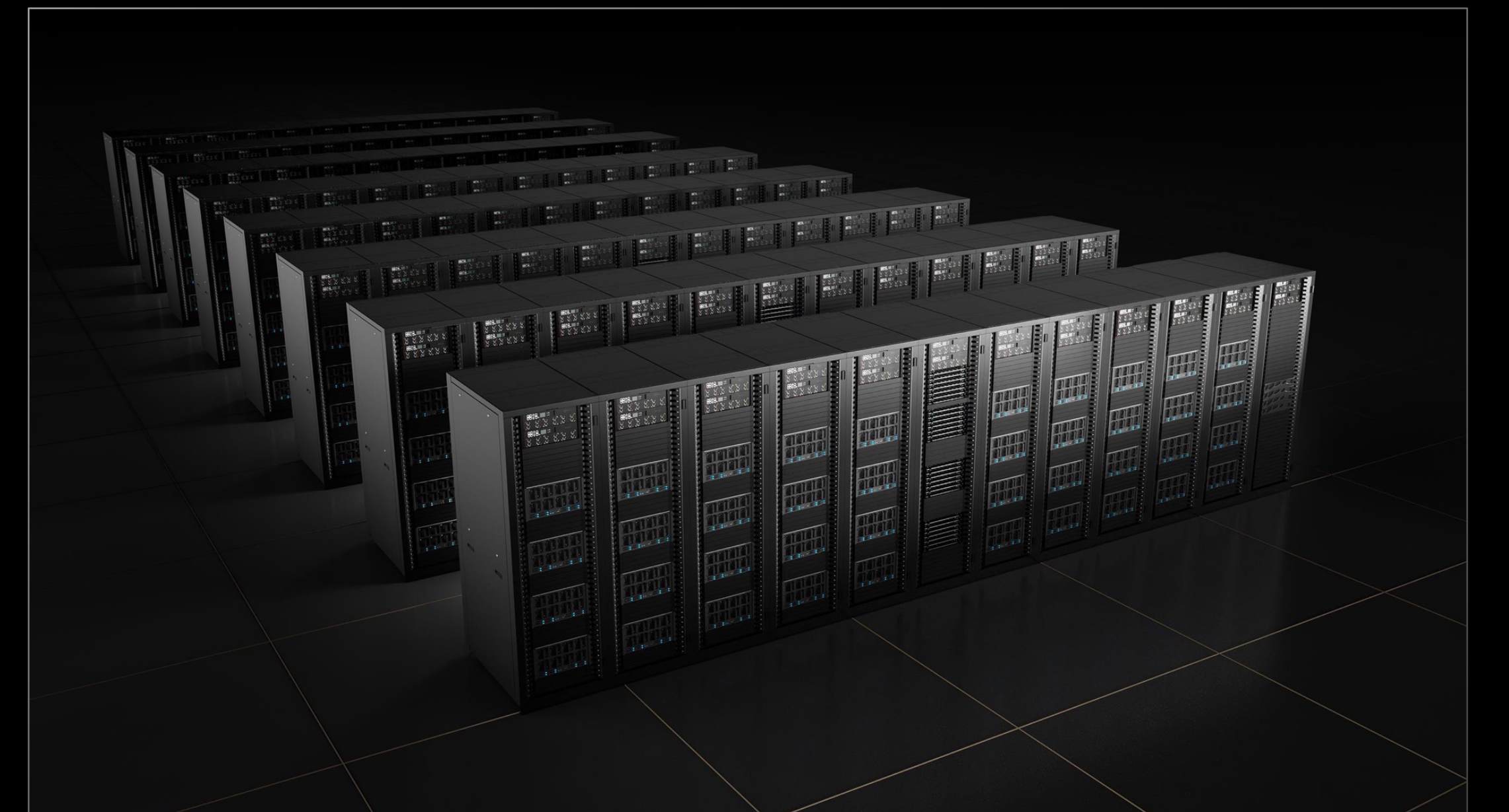
Multi-node NVLink/NVSwitch Infiniband
