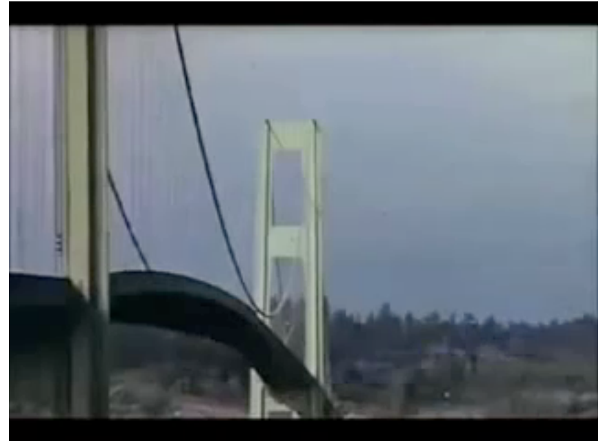
1940 Tacoma Narrows bridge collapse in 40 mph wind
